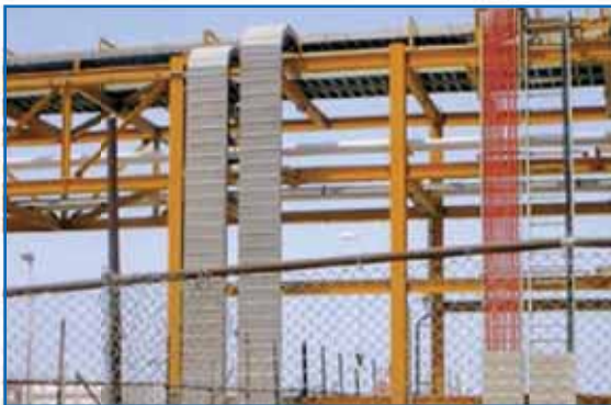
FRP Cable Ladder For Gas Processing Plant
