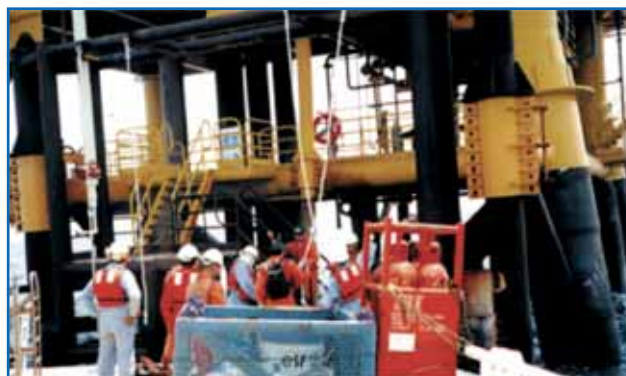
Installation Of FRP Grating On Offshore Platform (Brunei)
